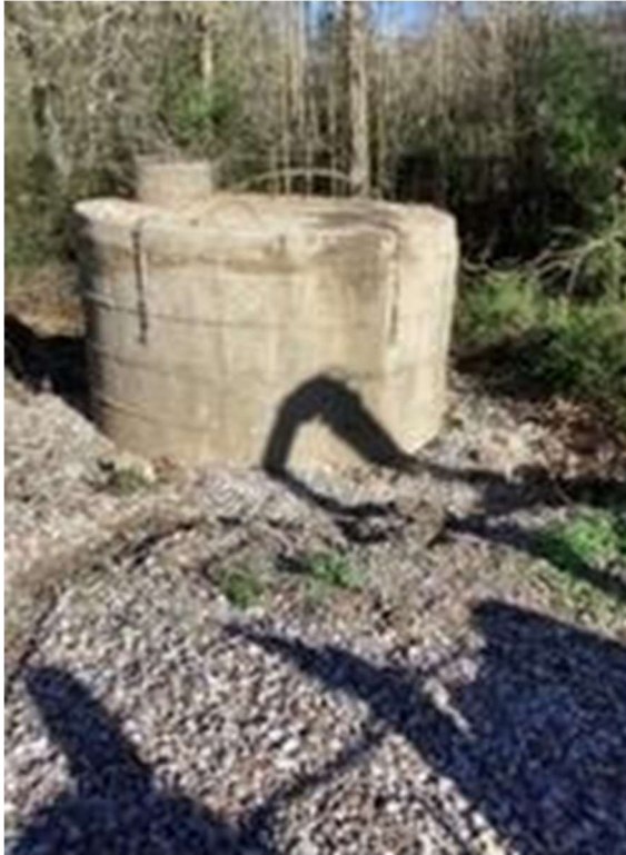
Manhole 1865 - 352 Fontana Road Before Cleanup
