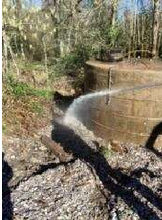
Manhole 1865 - 352 Fontana Road During Cleanup
