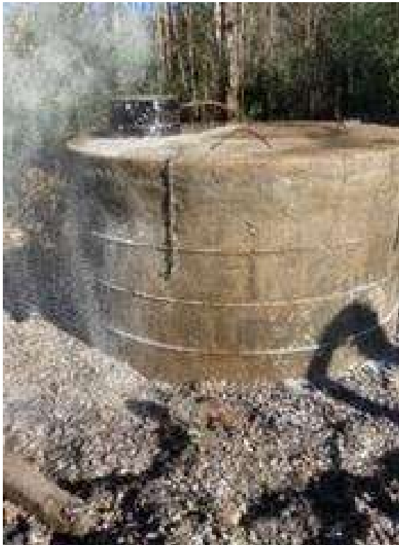
Manhole 1865 - 352 Fontana Road During Cleanup
